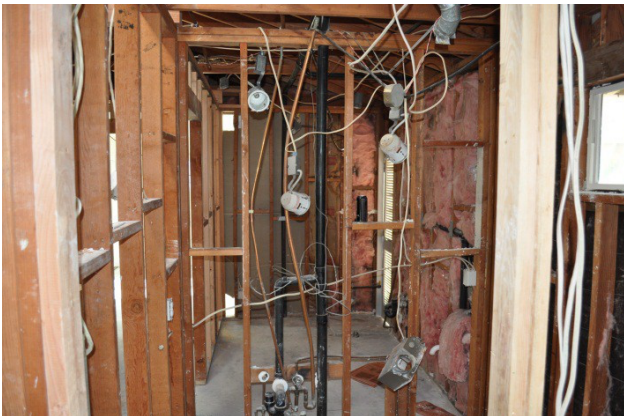
Typical bathroom renovation requiring the complete electrical and mechanical upgrades.
