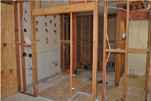
Typical bathroom renovation.
