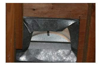
Above is an exterior and interior view of a screened vent installation. Note the ¼" screen. Eaves and Cornices, openings on the underside of eaves and cornices are not approved.
