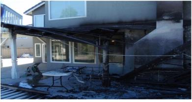
The walking surface material of decks, porches, balconies and stairs located in the VHFHSZ and Ember Zone 2 shall comply with the requirements of this section when any portion of such surface is within 10 feet of the building.
