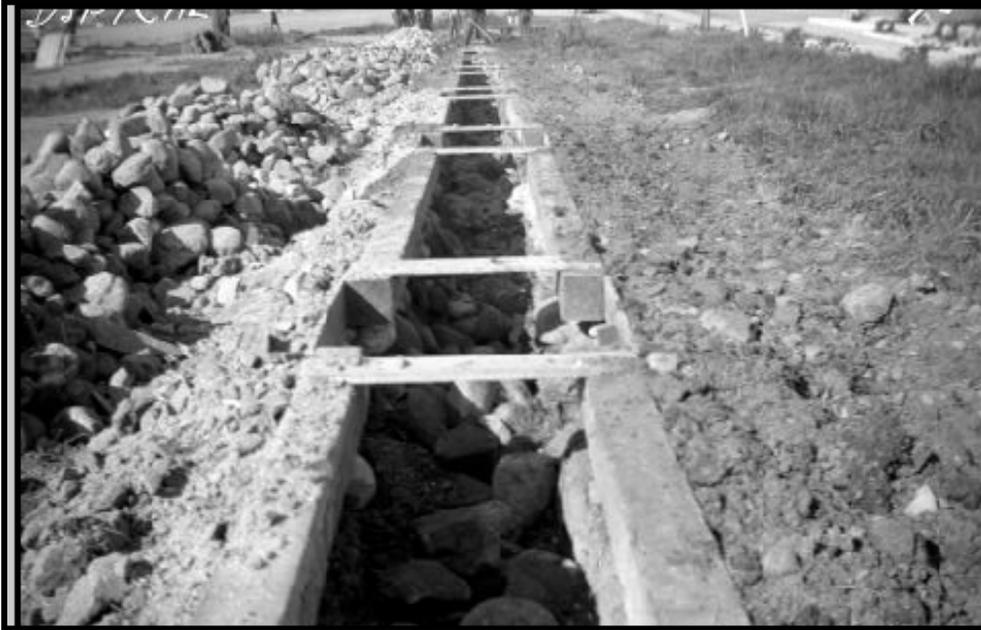
Cobblestone Foundation and Footing Framing Wall Trench
