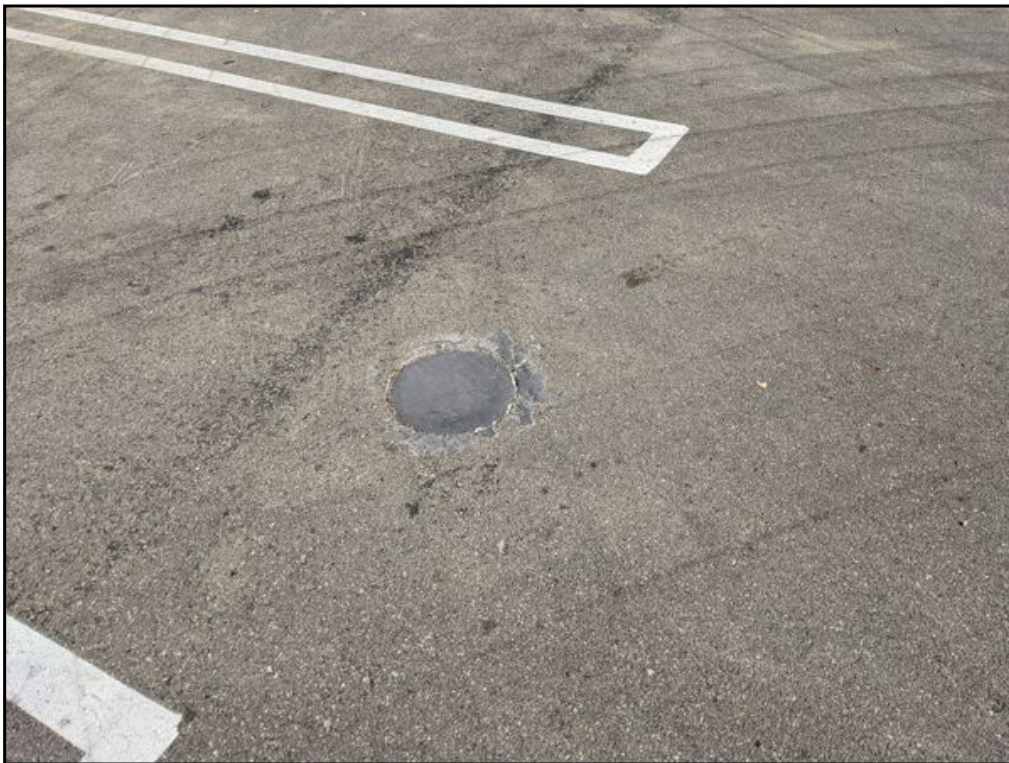
6 : Possible abandoned and plugged monitoring well near hotel building.
