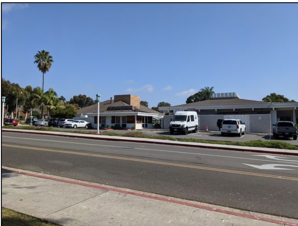
32 : East adjacent commercial buildings.
