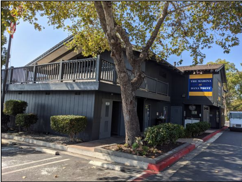
13 : On-site boater service building located at 34555 Casitas Place.
