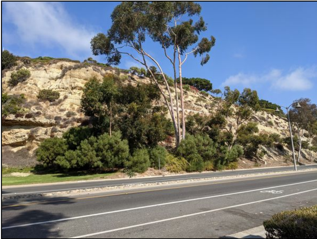
31 : North adjacent earthen slope.
