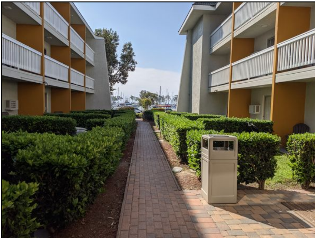
4 : Courtyard area at on-site hotel.
