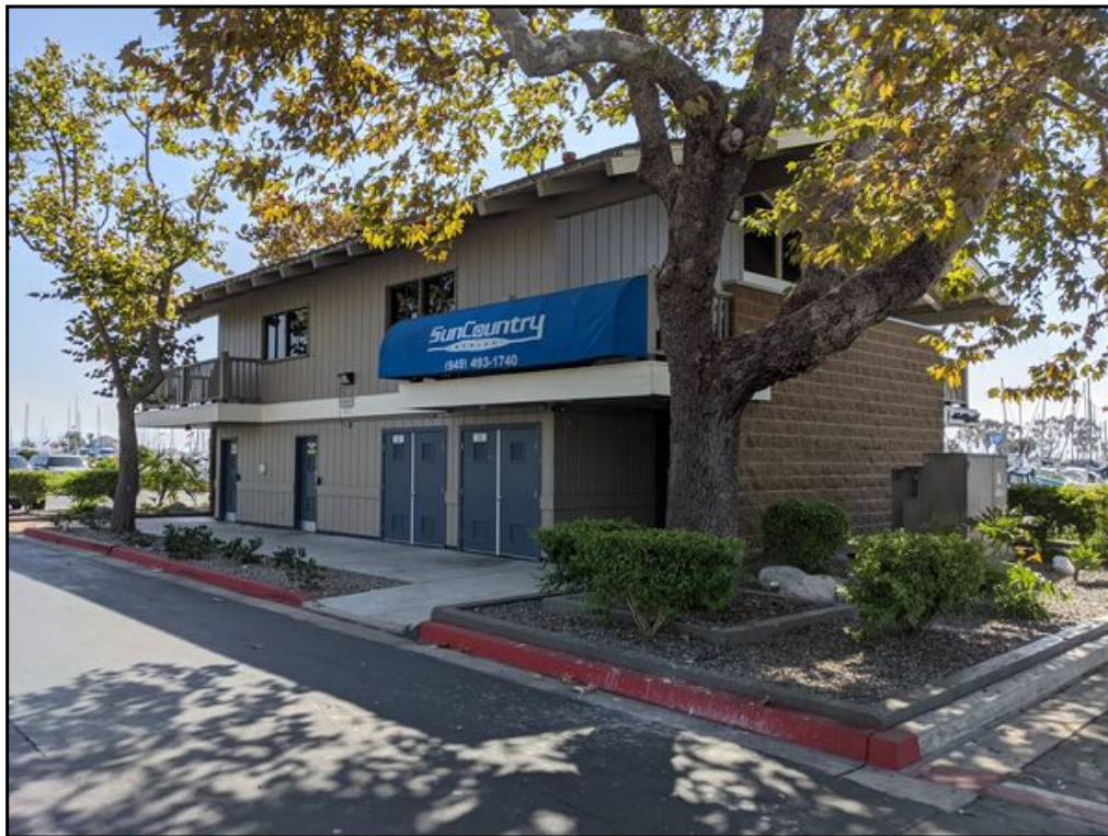
8 : On-site boater service building located at 34553 Casitas Place.
