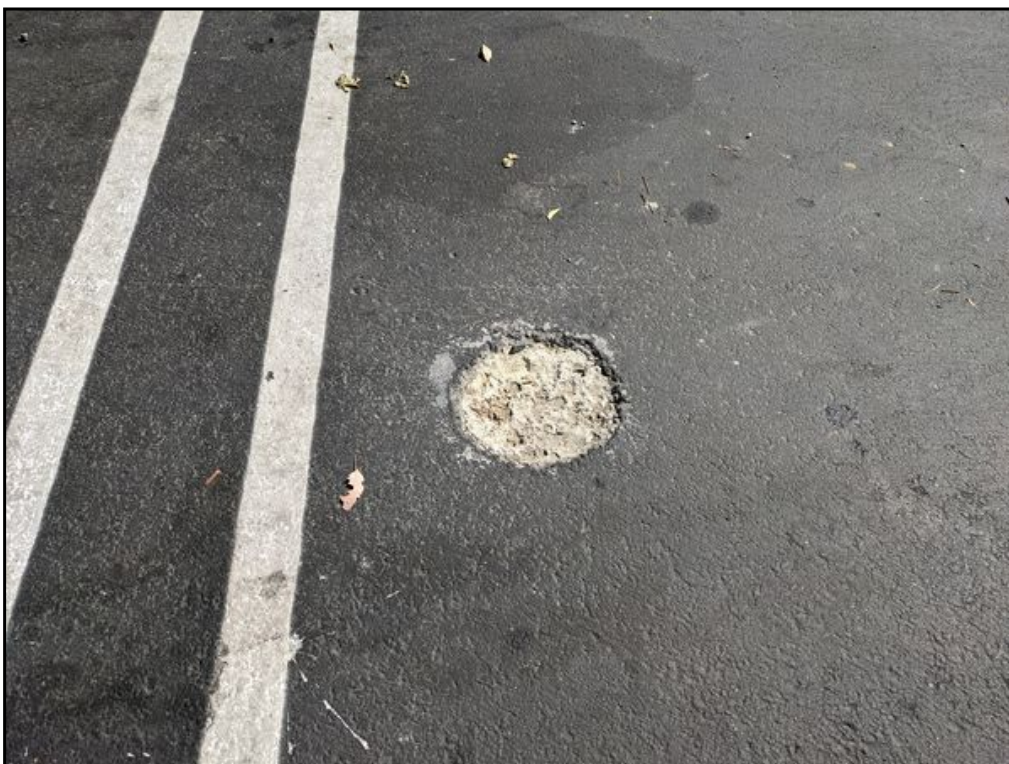
12 : Possible abandoned and plugged monitoring well in parking lot on south side of the site.
