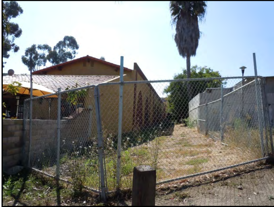
Photograph 3. North side of the hotel (the project site).
