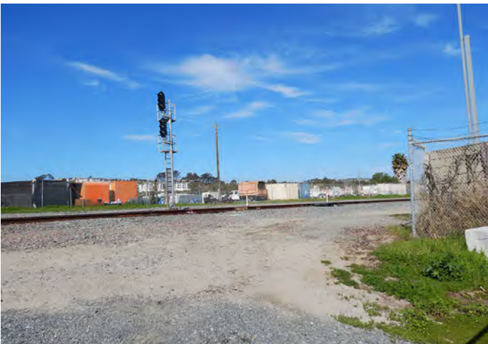
Western view of the Southern California Regional Rail Authority (SCRRA)/Orange County Transportation Authority (OCTA) railroad right-of-way to the west of the project site.
