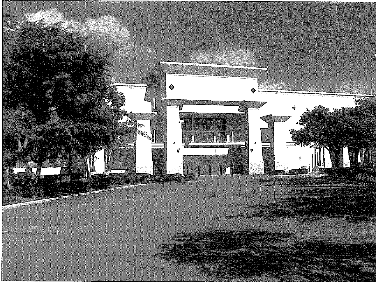
This is the former Expo Center on Rancho Niguel Road in Laguna Niguel. It is available and would be an ideal off-site location for the SSBC to purchase.
