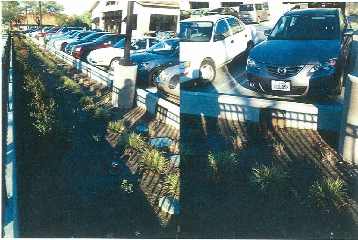
Storm Water Planters
