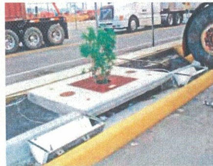
Filterra® monitoring unit at an industrial port.
