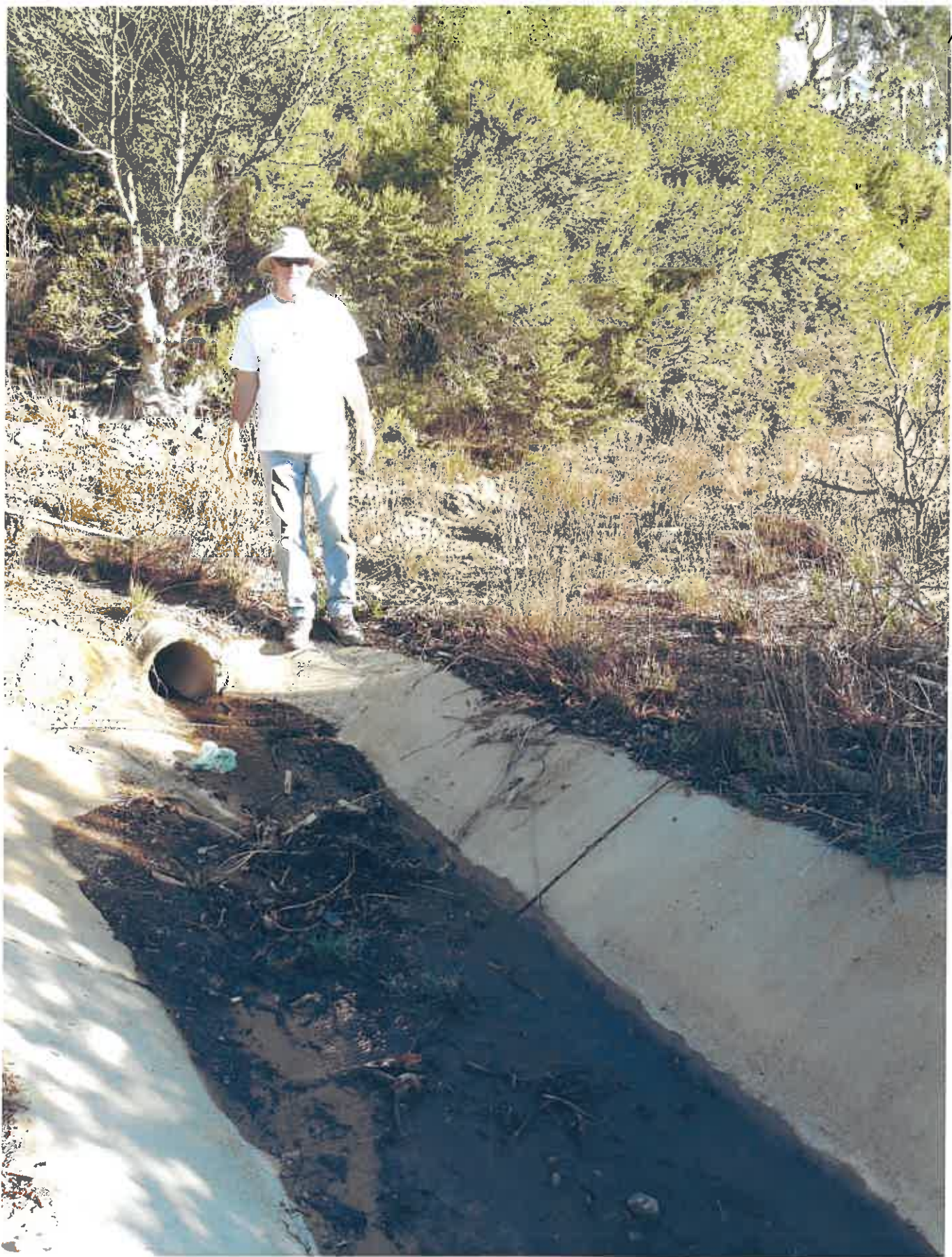
South Shores Church (SSC) southeast drainage to detention basin: Approx. 3.5 acres per DEIR Report
