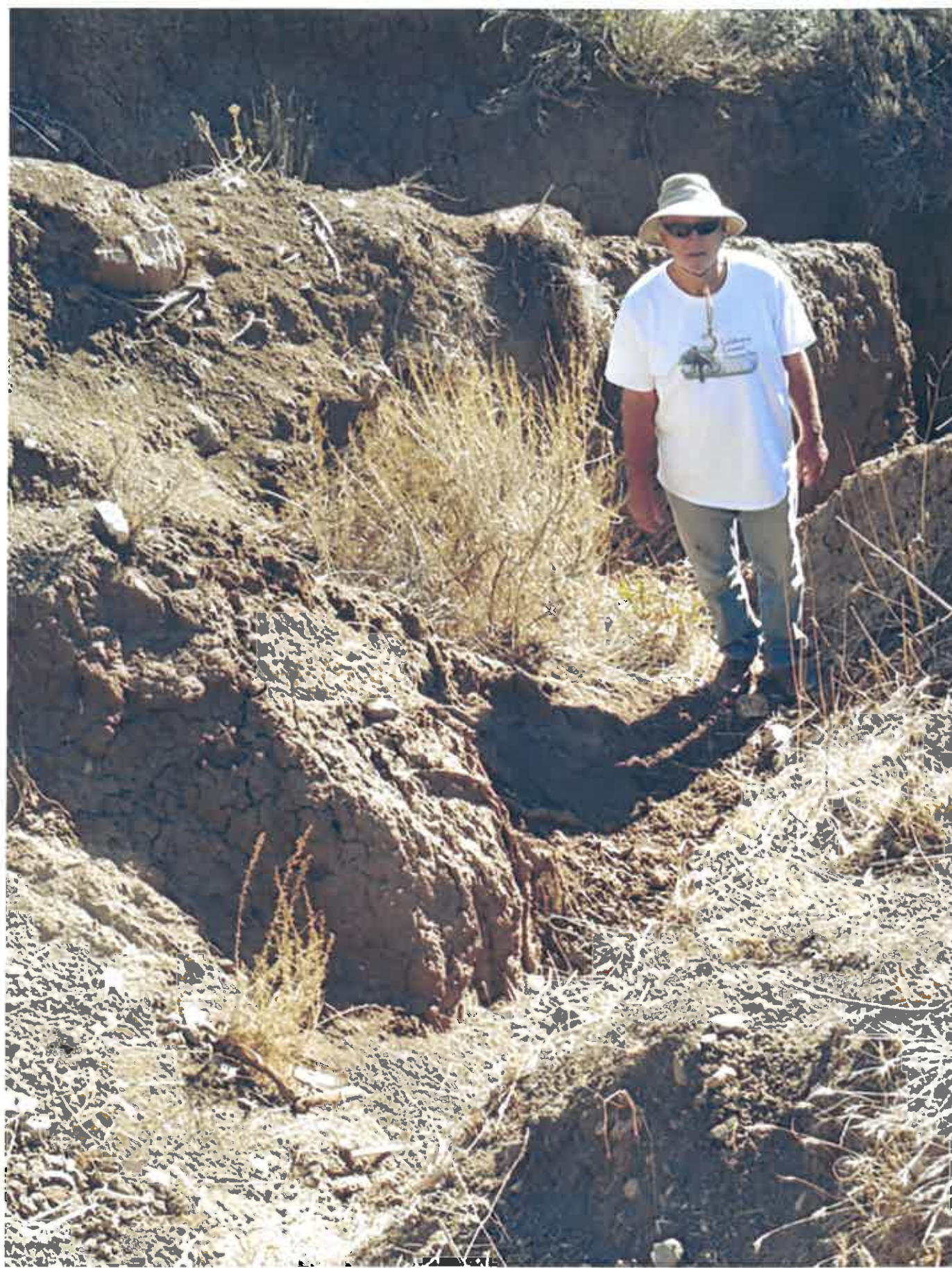
Gully now 20 feet deep, 40 feet wide, 200 feet long: Due to erosion, no v-ditch or detention basin maintenance
