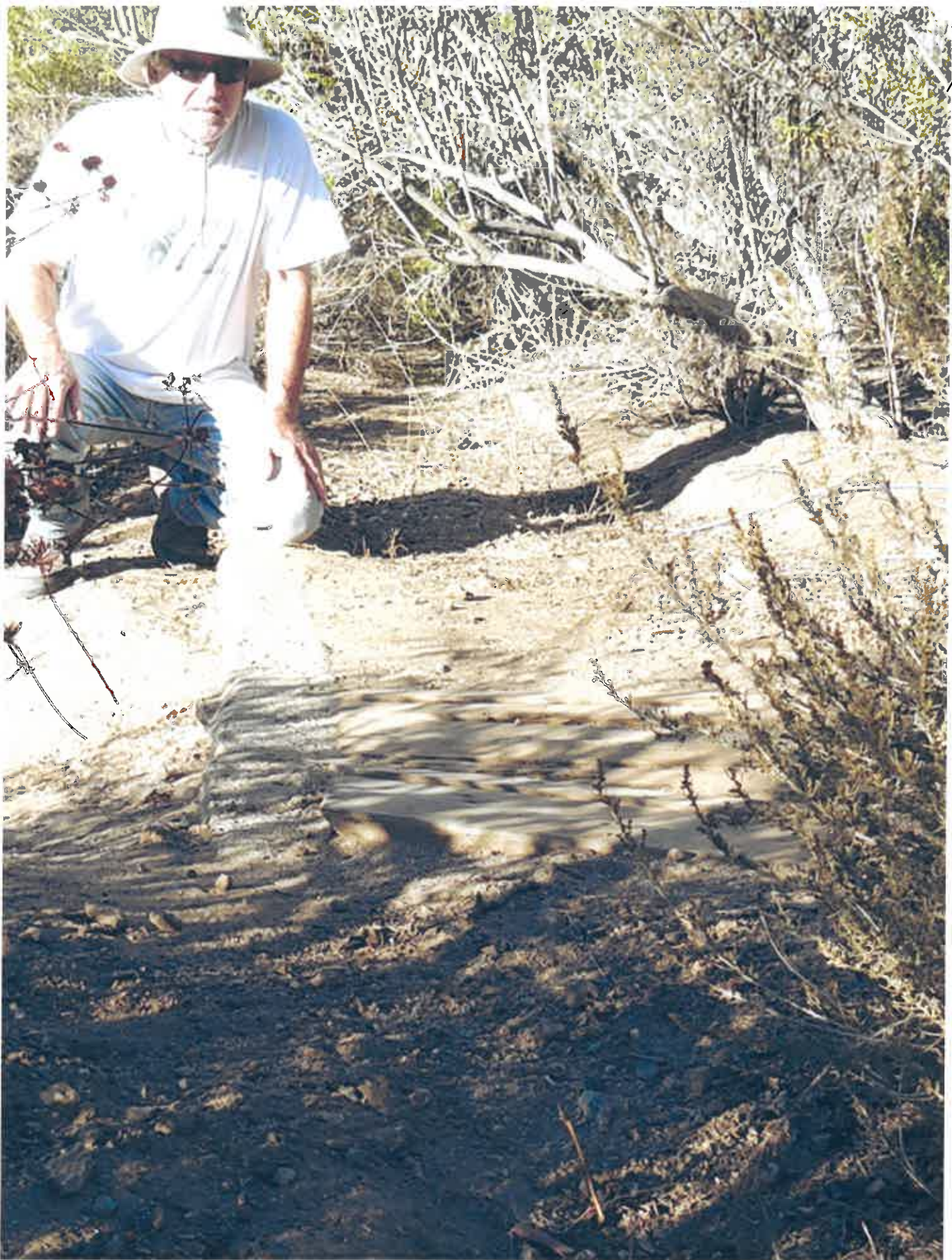
V-ditch from detention basin: Buried.
