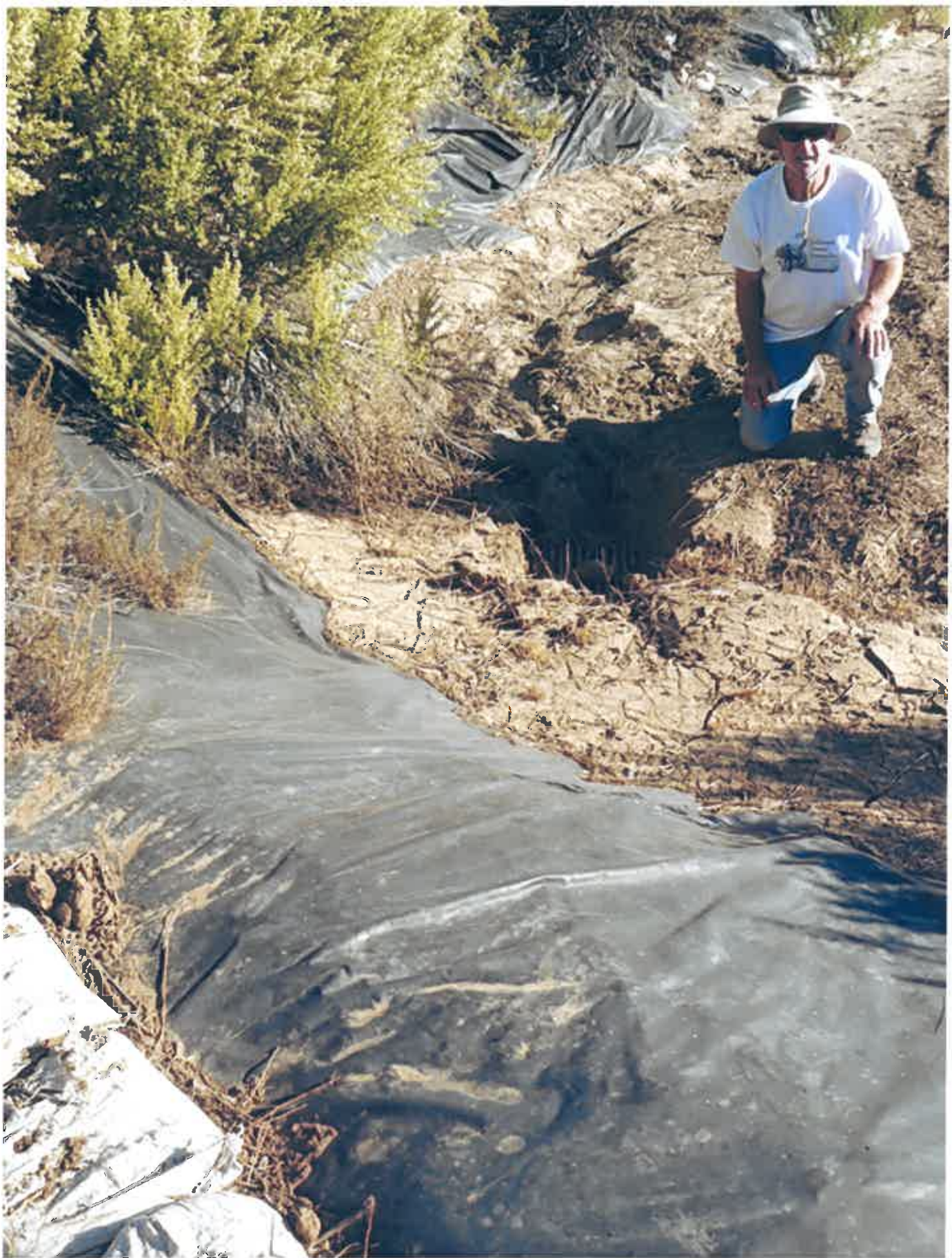
Salt Creek Corridor Trail storm drain intake perimeter buried under sediment near Pointe Monarch trailhead.
