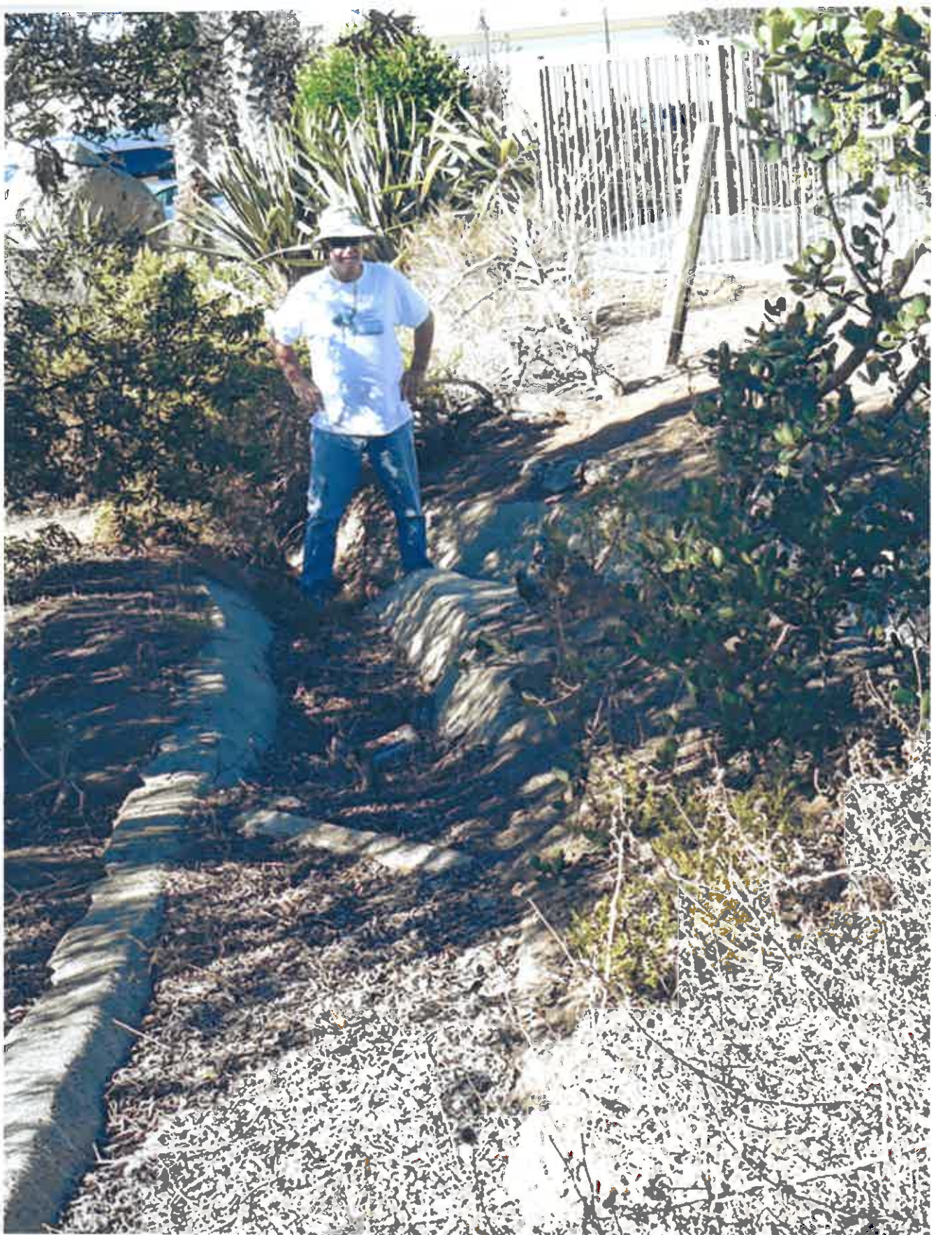
V-ditche confluence near Pointe Monarch: Left side in photo s ESA drainage, right side source is Monarch Beach Villa HOA v-ditch
