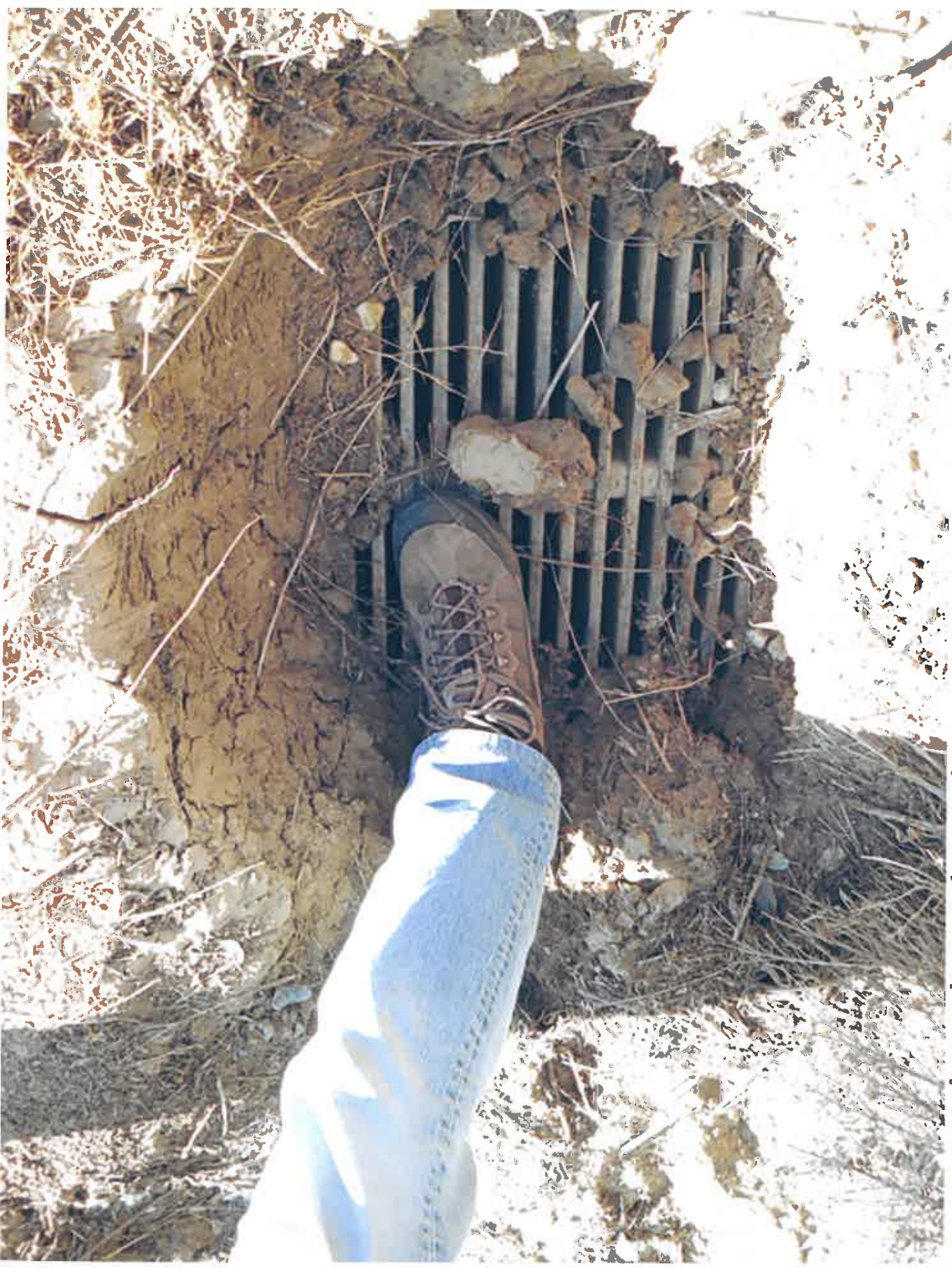
Salt Creek Corridor Trail storm drain intake near Pointe Monarch.
