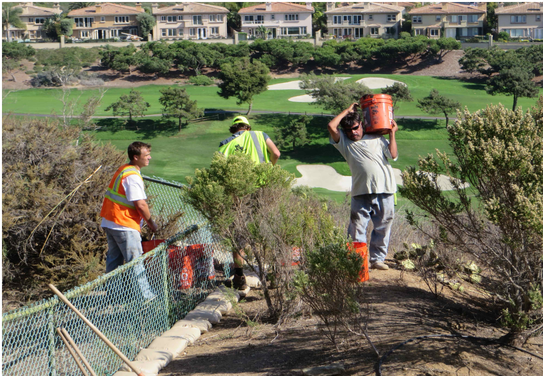
October 20, 2014. View of Applicant's employees clearing percolation basin.
