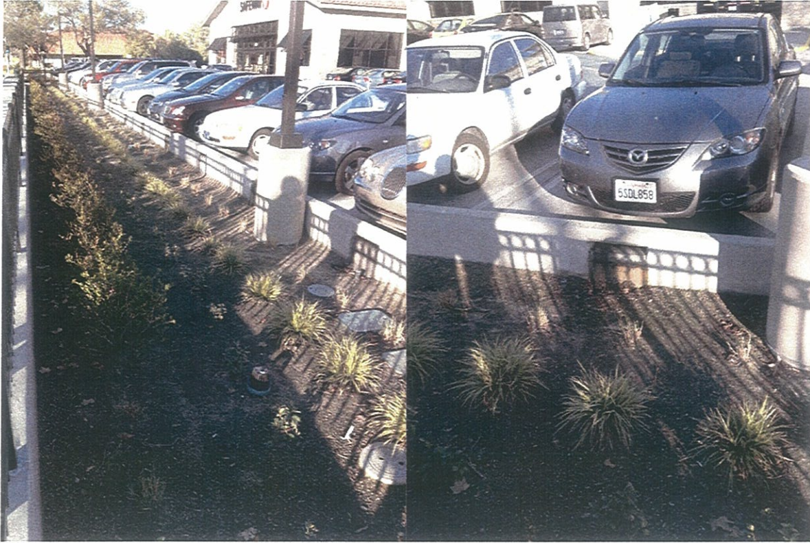
Storm Water Planters
