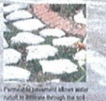
Permeable pavement allows water runoff to infiltrate through the soil and prevents road pollutants from reaching the storm drain system.
