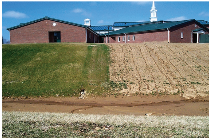
Figure 16. Seeding is an effective BMP that can be used to temporarily or permanently stabilize disturbed areas.
