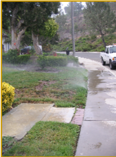
Adjusting misaligned and leaky spray heads can save 20 gallons a minute!
